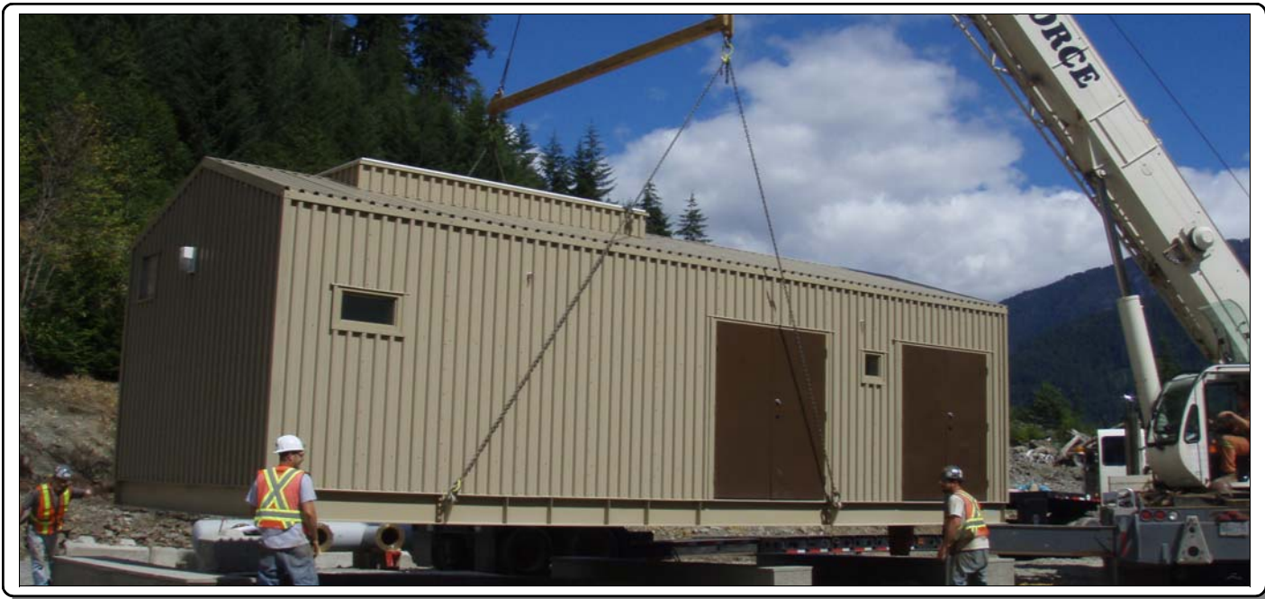
Prefab Pump House and Installation
