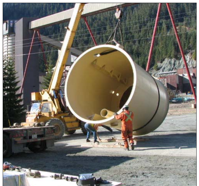
Installation of Mine Processing Equipment
